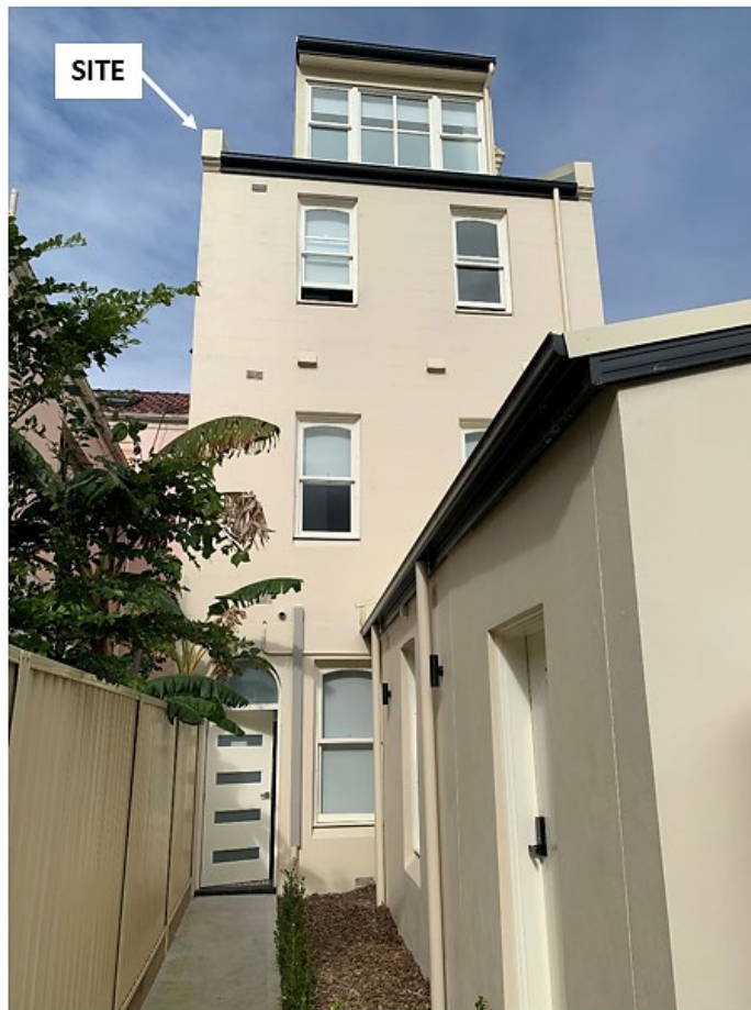
northwest elevation and rear wing of existing terrace
